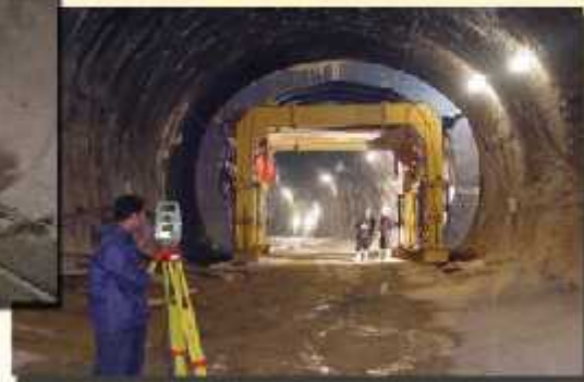
Tehran Metro line No. 1 – Tunnel of Section I and S1 station
